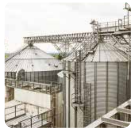
Storage Grain Silos / Warehousing
